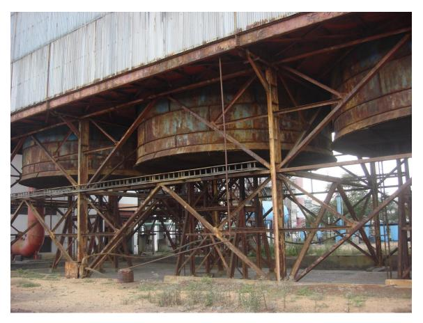
Figure 35, Condensers of Hyderabad RDF-WTE Plant, Elikatta
