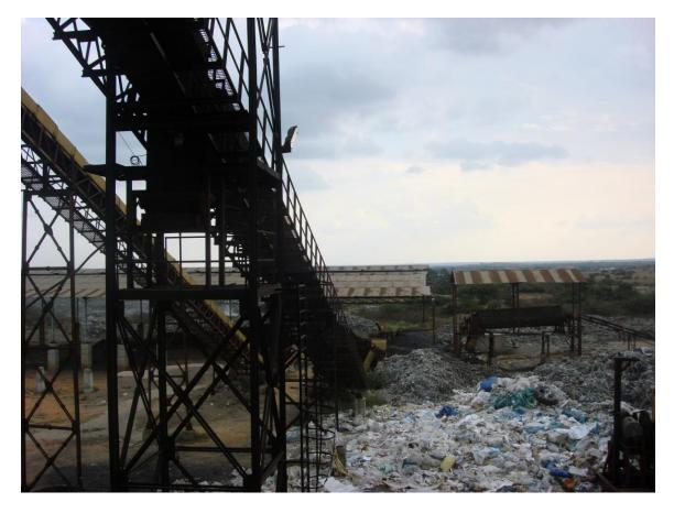
Figure 34, Conveyor Belt for Feeding RDF into the WTE Boiler, Hyderabad RDF-WTE Plant, Elikatta
